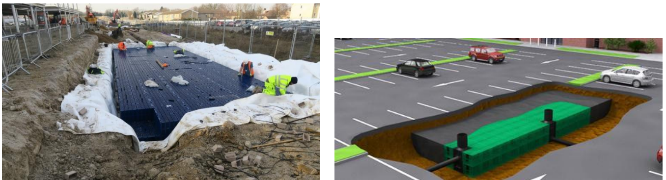
Figure 4-10: Geo-cellular attenuation tank/soakaway
